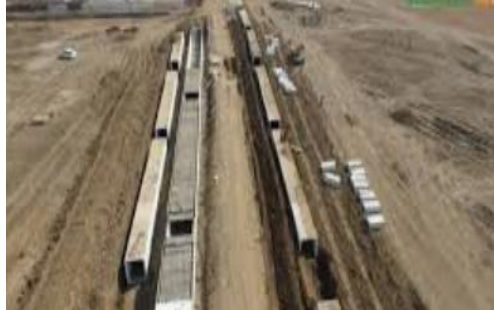
Drainage network construction
